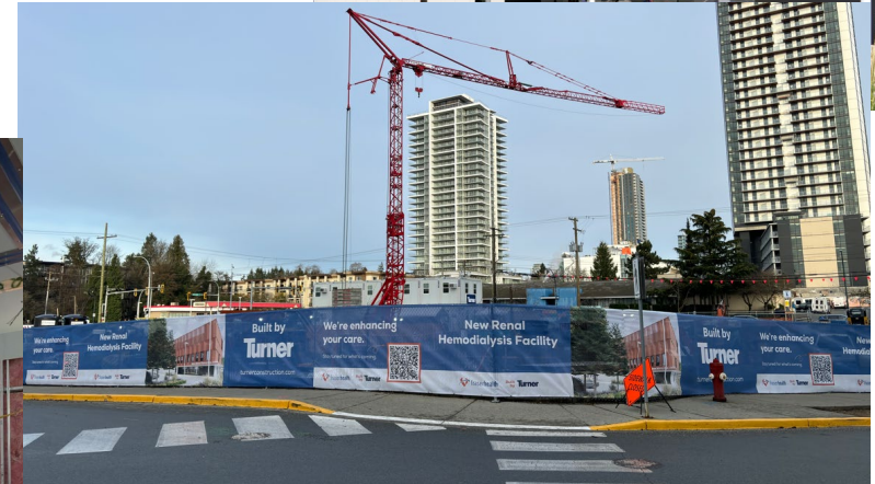
Renal Building construction
