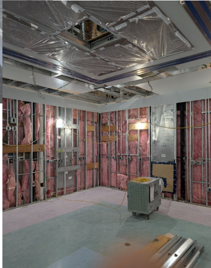
Operating Rooms Renovation
