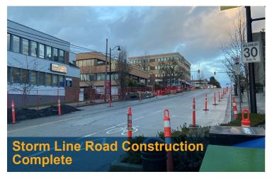
In Fall 2020, we installed a new storm line down the centre of East Columbia St. as part of the City of New Westminster's storm line sewer separation program.
