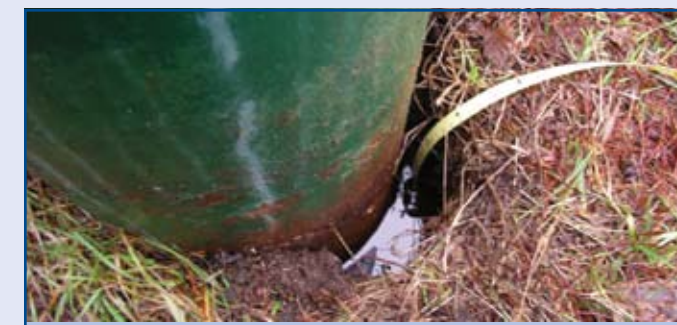
Well with gap between casing and ground – no surface seal
