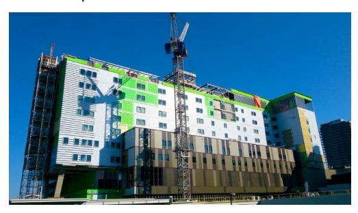
We are making great progress on both the interior and exterior of the Jim Pattison Acute Care Tower. Work is underway on all floors and our construction partner, EllisDon, is installing the new modular heliport on the roof. They are also installing a new retaining wall with a sidewalk to create a multi-use path by the hospital service lane. The sidewalk on the east side of the hospital will be closed until late November 2023. Thanks for your patience during this work. Read more.
